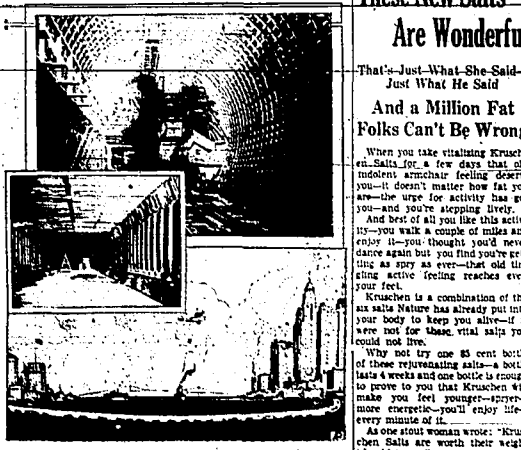
(left) was built in huge sections (top) and sunk under surface to link United States and Canada (below).
