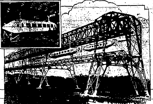
An experimental railplane system has been built in Scotland and will be tested in July. At the upper left is a railplane coach under construction in railroad shops.
