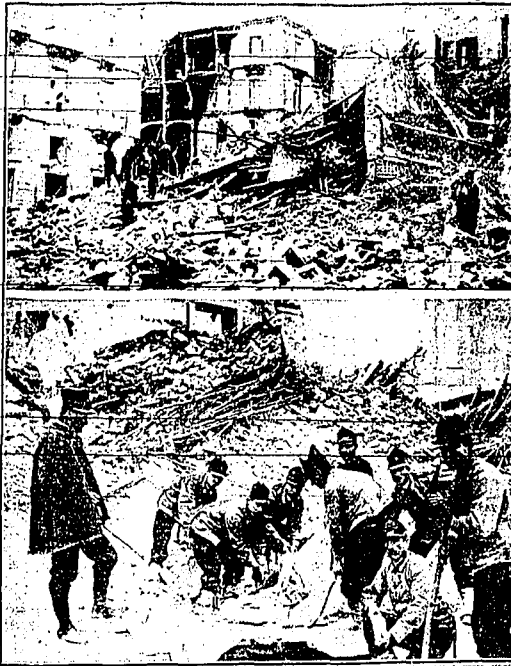
HUNDREDS WERE KILLED when earthquakes devastated towns in southern Italy. The disaster caused the most widespread death and devastation since the Messina earthquake of 1908 when 75,000 persons were killed. The pictures above were made following the Messina disaster. Upper picture shows buildings reduced to rubble. Below soldiers removing body of victim from wreckage. (AP) Photo.
