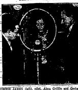
IIMMIE IAMES (16f1), pilot, Alma Griffin and Gerhar Fisher aboard a plane over Los Angeles, test a new radi direction finder by which a pilot can tune in on a radi atation and be guided to it by the finder indicator. The device was designed by Fisher and perfected by Her bert Hover, in.—(F) Fisher.
