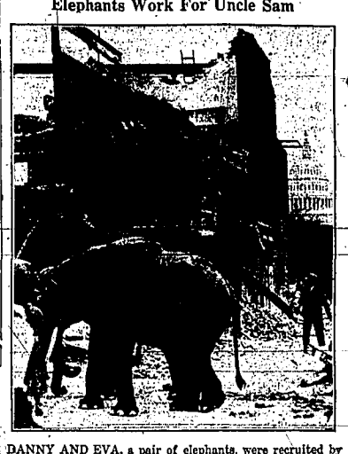
Elephants Work For Uncle Sam DANNY AND EVA, a pair of elephants, were recruited by Washington authorities to help pull down buildings on Pennsylvania avenue...
