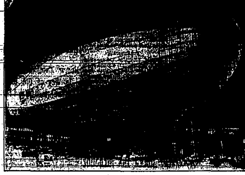
THE HUGE UNITED STATES Ship Macon, sister ship of the giant Akron, is virtually completed. All fuel tanks have been installed, two of the four fins are in place, and instruments in the control car soon will be installed. After it is finished in March and accepted by the navy, it will be based at Sunnyvale, California.—AP Photo.
