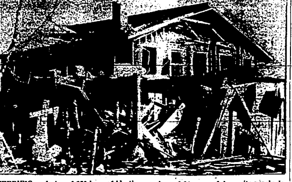
A TERRIFIC explosion of 250 kegs of blasting powder and 20 cases of dynamite nearly destroyed Helenwood, Tennessee. Fifty homes and buildings were destroyed or damaged, seven persons injured and 75 made homeless by the blast. This picture is typical of the destruction caused. (P) Photo.
