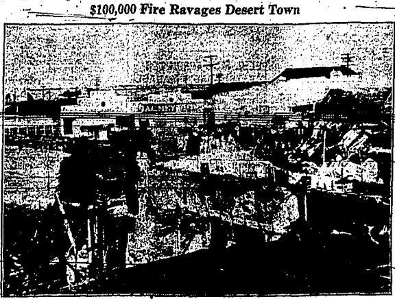
$100,000 Fire Ravages Desert Town FIRE, fanned by a hot desert wind, did $100,000 damage in the Mojave desert town of Lancaster, California. Five buildings in the heart of the business district were destroyed. Part of the ruins is shown above.—(A7) Photo.
