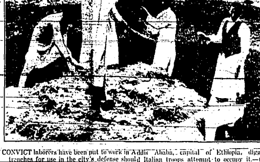
CONVICT laborers have been put to work in Adiga, capital of Ethiopia, digging trenches for use in the city's defense should Italian troops attempt to occupy it. (AP-Paramount News-Photos)
