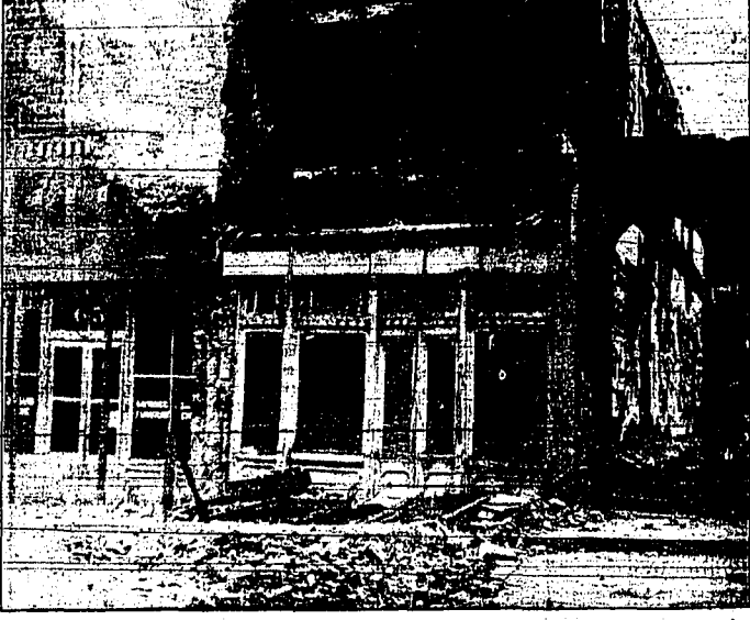
DAYE HARRIS, a Negro, was crushed to death when this building collapsed in Helena, Montana. One other person was known to be dead and nearly a score injured in the severe earth shock which hit the Montana capital...
