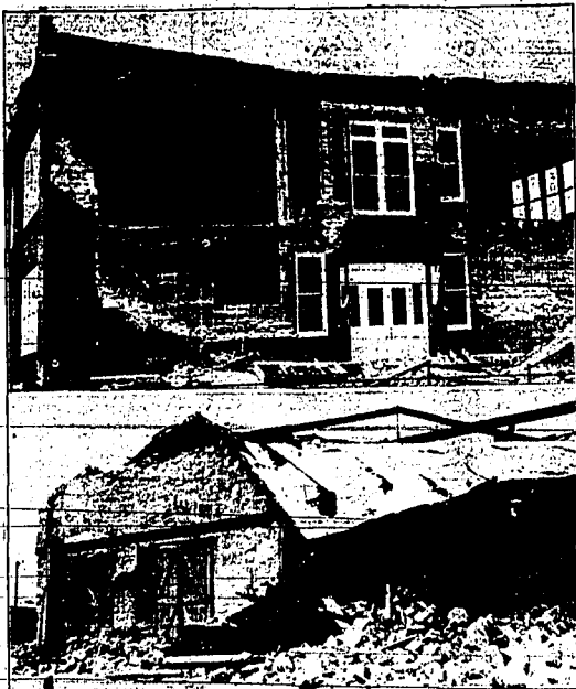
THE capital city of Montana was violently jolted in a second series of earthquakes which added two more deaths to the quake toll. Top: Wreckage of the Bryant grade school in Helena and (lower) a damaged warehouse. (AP Photo).
