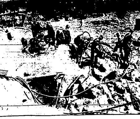
A JACKHAMMER crew at work on the bedrock of the west excavation of the Grand Coulee dam on the Columbia river in Washington. They are drilling preparatory to placing a blast that will prepare the rock for the dam's foundation. (AP Photo).
