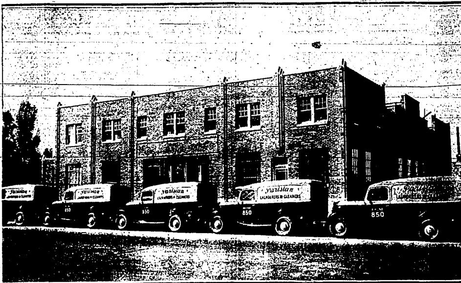
Pictured above is the newly completed home of the Parisian Laundry and Dry Cleaners. Designed from the start and built by expert laundrymen this splendid $100,000 structure represents the last word in modern machinery and equipment to economically and satisfactorily serve the needs of this community. When operating at full capacity this institution will furnish steady employment for 60 or 65 people.
