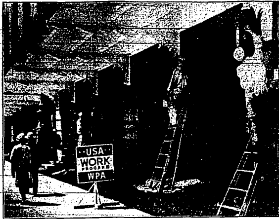
THE $300,000 for the job of refurbishing the Cleveland convention hall for the Republican gathering came mostly from federal relief funds. Hence this WPA sign as workmen put the final coat of white paint on the marquee. (AP) Photo.
