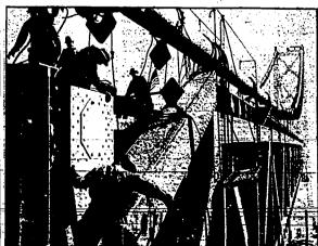
are workmen placing in position the last section of steel to complete the superstruc-e of the huge San Francisco-Oakland bay bridge. The beam is shown being raised in-ts diagonal position. With completion of this phase of the work, only the flooring of double traffic decks remained to be done—(P) Photo.
