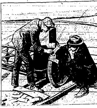
A novel method of testing automobile tires, employed by a Denver manufacturer... The tire is attached, through the open hubways...
