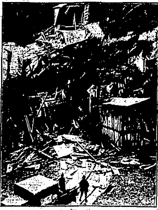
TWO MEN scramble to safety, one only slightly hurt and the other unscathed when a landslide demolished a power house wall at the Fugate Sound Power and Light Co. at Ellettsville, Wash. This picture shows the shattered remains of the expensive machinery and buildings.
