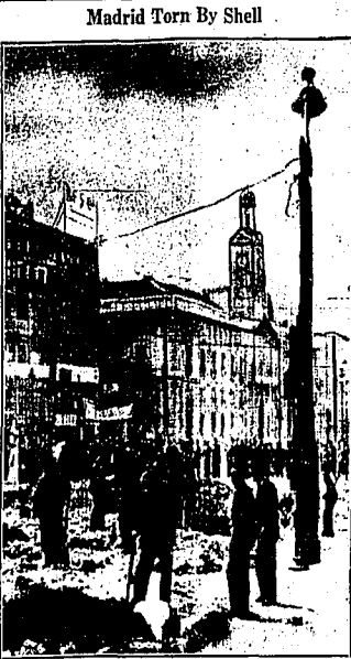
Madrid Torn By Shell
