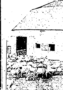
Fourteen-sided barn 18' 0" in diameter and has a 12-foot slope to the top.
