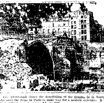
Photograph shows the demolition of the famous bridge in Paris...
