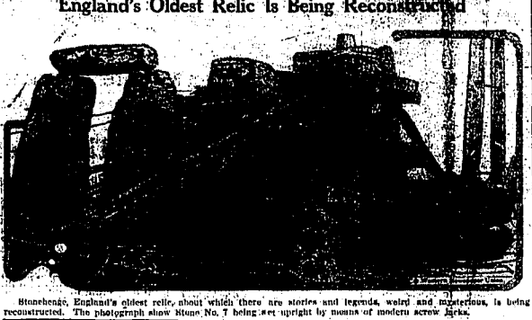
Stonehenge, England's oldest relic, about which there are stories and legends, being reconstructed. The photograph shows Stone No. 7 being set upright by means of modern screw jacks.
