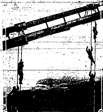
These men are cutting ditches 122 feet in the air because they have just completed the span of the new suspension bridge across the Hudson river at Peekskill, N. Y. It is the highest and longest suspension bridge in the world—its main span is 1,615 feet long—its towers are 455 feet high.
