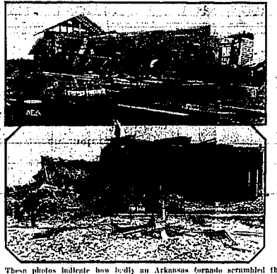
These photos indicate that today an Arkansas tornado scrawled the town of Green Forest the other day. The storm killed a score. The upper picture shows what was left of the home of Will Tate. Below is the wreckage of the town school.
