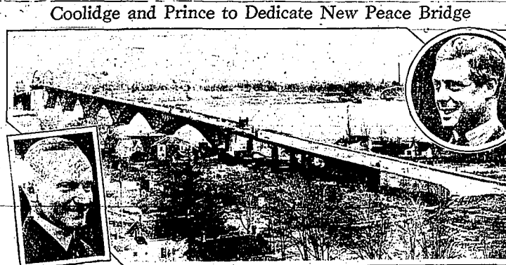
The new Peace bridge, connecting Buffalo, N. Y., and Fort Erie, Canada, is pictured above. It is nearly complete and is to be dedicated in May by President Coolidge and the Prince of Wales. The span is dedicated to the 100 years of peace between the United States and Canada and as a reminder that no fortifications exist on either side of the border from coast to coast.
