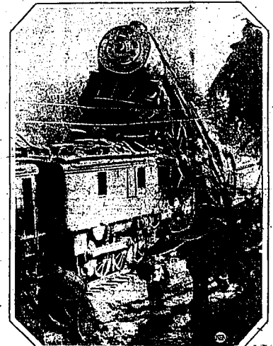
This remarkable picture, taken following a train wreck on the Virginia railroad near Inglewood, Va., in which two were killed and 20 injured, shows a locomotive atop an electric motor. The two trains crashed head on. Removing the engine gave workers a problem.
