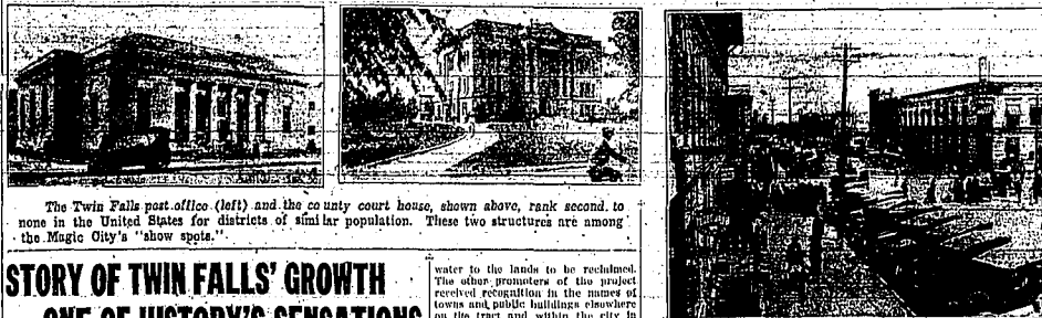
The Twin Falls post office (left) and the county court house, shown above, rank second to none in the United States for districts of similar population. These two structures are among the Magic City's "show spots."
