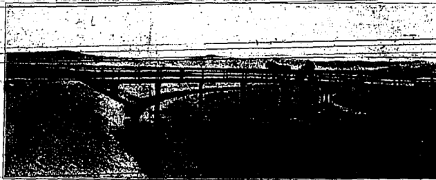
Main Canal of the Twin Falls system, as it appears today, carrying about one-third of the normal flow of water. This canal was filled to the brim last spring by water which flowed down in the coulees from the mountains to the southward. The canal is 120 feet wide at the top and 80 feet wide at the bottom. It is constructed to carry 10 feet of water.
