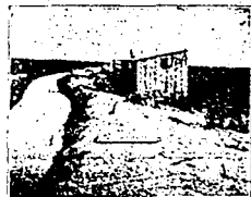
Mr. Provevsky's Ditch, with a Side View of the "Shack."
