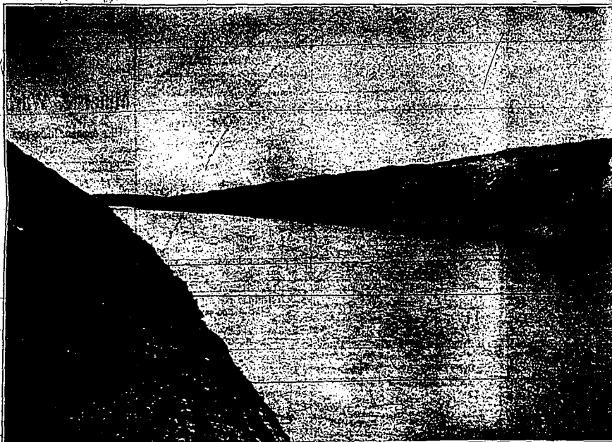
Main canal, Twin Falls North Side Land & Water Co., in the big cut, two miles from Milner dam. This cut is one and one-half miles long, with a maximum depth of 24 feet. The canal in the cut is 60 feet wide on the bottom. The runways in the sides of the right bank are wide enough for teams and were used in hauling out the dirt. Approximately 400,000 square yards of earth were taken from this cut. In no place was rock encountered. The banks of the canal show the depth of soil.
