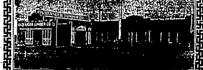
Office and yard: Shoshone Street and O. & L. R. R. Track.
