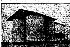
These bins were built by us three years ago for the Corinne Milling & Elevator Co., Corinne, Utah, and have given complete satisfaction. Each bin has a capacity of about 5,000 bushels of grain.
