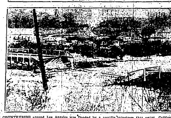
THE COUNTRYSIDE around Los Angeles was flooded by a terrific rainstorm that swept California. This scene shows how the auto bridge on the road between Los Angeles and Glendale was washed down by the tempest.
