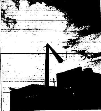
Friday's storm in Twin Falls was too much for the smokestack at the Parlan laundry, 712 Main avenue south. The above photo shows what happened to the smokestack. No one was injured and operations of the laundry were not curtailed. Repair work was under way Saturday. (Staff photo-enlarging)
