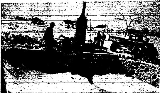
Charles W. Blat, city engineer at Gooding, is shown above as he uses steam to clear ice from the Nevada street bridge in Gooding. Clarence Moore is in charge of the boiler used to generate steam. Residents of Gooding are doing everything possible to clear channels in anticipation of high water and ice jams in the local future. (Photo by Letha Teasler—staff engraving)
