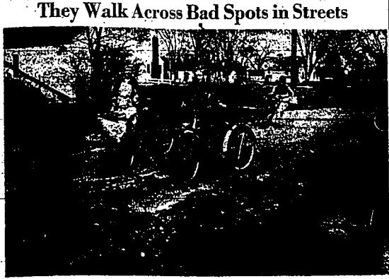
Children riding bicycles are shown above as they push their vehicles across a rutted spot on Elbow street between Blue Lakes boulevard north and Lincoln street. Similar spots are developing almost overnight on Twin Falls streets as frost leaves the ground. Some spots have become so hazardous they have been blocked off. Pushing their bicycles in the above photo are Levere and Doug Emrick, the children of Mr. and Mrs. Cliff Emrick, 183 Taylor street. (Photo by Herb Kinnear-staff engraving)
