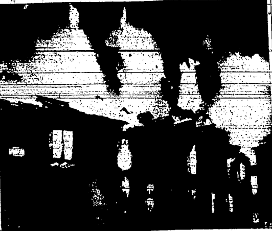
View of St. Andrew's hospital at height of fire where at least 72 persons, including 12 newborn infants, the American Red Cross reported, were dead or missing in the night fire which rapidly consumed the building at Effingham, Ill. (AP wirephoto)
