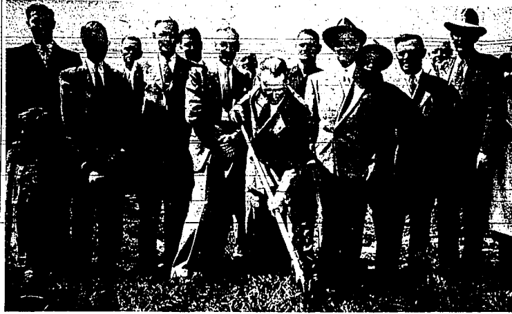
DeWitt H. Young, chairman of the board of county commissioners, today presided over the first shovel full of dirt for the new Twin Falls county hospital during a ceremony Monday morning.
