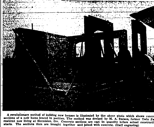
A revolutionary method of building new homes is illustrated by the above photo which shows concrete sections of a new home braced in position. The method was developed by M. A. Burson, former Twin Falls resident, now living at Hermiston, Ore. Concrete sections are cast in quantity before actual construction starts. The sections then are brought together and joined with concrete. (Staff engraving)
