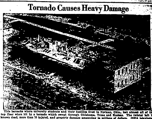
This barracks where university students and their families lived in Norman, Okla., lost almost all of the top floor when hit by a tornado which swept through Oklahoma, Texas and Kansas. The twisted left 10 known dead, more than 10 injured, and property damage amounting to millions of dollars. (NEA telephoto)
