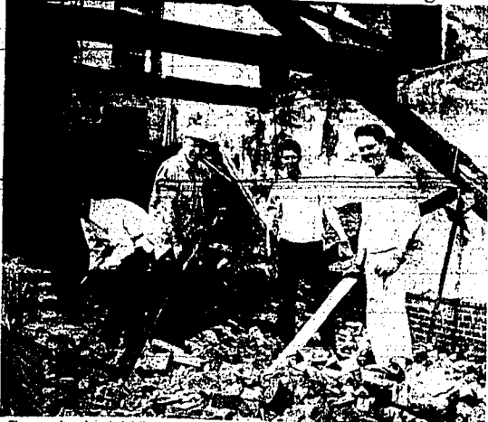
The crew above has started the work of tearing down and remodeling old Swagson hall on the campus of Southern Idaho College of Education, Albion, badly burned during the summer of 1947. Recent appropriation by the state legislature permits the present activity and portions of the old building are expected to be remodeled and ready for classroom use by the fall term. (Photo by Edward Matthews—staff engraving.)
