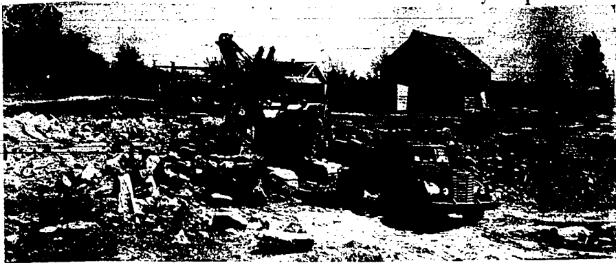
Tons of lava rock are being removed from the site of the new Twin Falls county hospital as work is rushed on the new structure. Photo at top shows power shovel loading trucks with rock broken by blasting. About 1,000 cubic yards of rock have been removed with another 2,000 cubic yards to be moved before the foundation of the building can be laid. In photo at bottom, carpenters are shown with stacks of lumber has been stacked at the site of the building, about 60,000 board feet will be used in the project. In background are the present buildings of the Twin Falls county hospital. (Photos by Joel Shulman—staff engravings)
