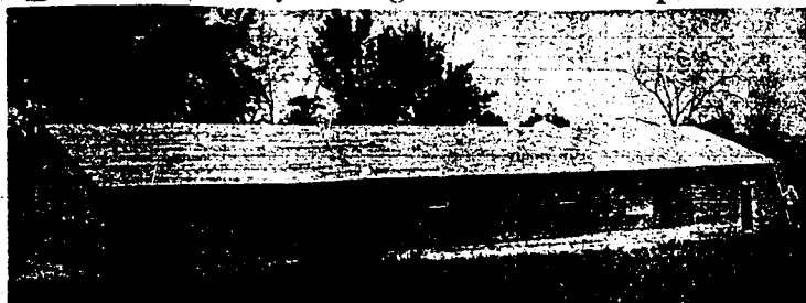
Construction work is nearing completion on the Twin Falls canning kitchen shown above. Equipment is expected to be installed in the building by July 1. Construction is financed by sale of common and preferred stock. (Staff photo-engraving)
