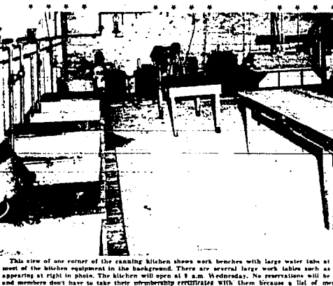
This view of one corner of the canning kitchen shows work benches with large water tubs at left and most of the kitchen equipment in the background. There are several large work tables such as the one appearing at right in photo. The kitchen will open at 8 a.m. Wednesday. No reservations will be required and members don't have to take their membership certificate with them because a list of members is kept in the office near the entrance to the building. (Staff photo-gravure.)
