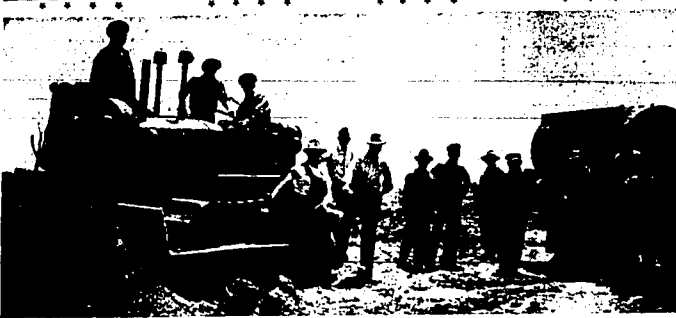
Eden residents and farmers are donating their time to build a road from Eden to Hunt across five miles of desert land. The work is being financed by donations. In photo at top, four Eden carpenters work on 12-foot bridge across the Jerome canal. They donate their services. Left to right are M. Schutte, Neal Mesnick, Herbert B. Schutte and Charles Hawley. In lower photo are a number of residents of the Eden area who are working on the project. Left to right are T. Walters, Herman Schutte, Martin Volter, Charles Hawley, Guy Lattimer, Vernon Lauce, A. G. Varner, M. Schutte, Jas. Hand, Neal Mesnick, Herbert B. Schutte, Fred Young and Bill Walters. Not present when the photo was taken was E. J. Davidson, past president of the Eden Edens club, who helped originate the idea for the road, a project of the Edens club. (Staff photo—engravings)
