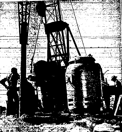
What is believed to be among the largest deep well irrigation pumps ever made has been installed on dry land north of Marsart owned by Julia Clawson. The pump, shown above, delivers 4,000 gallons of water per minute. It is rated as the horsepower of 1200 hp. It was installed under direction of the Idaho deep well irrigation pump he has installed. Several years ago Clawson, a former 6th Lake City newspaper man, bought 24,000 acres of dry land north of here. He has sunk five deep wells having a flow of 20,000 gallons per minute and uses a similar system to water parts of the 24,000 acres brought under cultivation last year. Other deep wells are being sited nearby. (Staff engraving)
