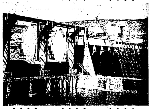
At top left is shown the west face of the dam being built near Bliss by the Morrison-Knudsen company for the Idaho Power company. In the foreground is part of the coffer dam which protects the installation while workers complete construction. On top right the west face of the dam is shown with the steel for the four huge gates which will control the flow of water through the structure. In the foreground is part of a mammoth walking crane which handles heavy machinery. In the center foreground are men working where one of the generators will be installed. Other workers are above of the "pile", an integral part of the installation. At bottom left is the east face of the dam, abutting two of the four gates and in the foreground is the concrete structure of the dam.
