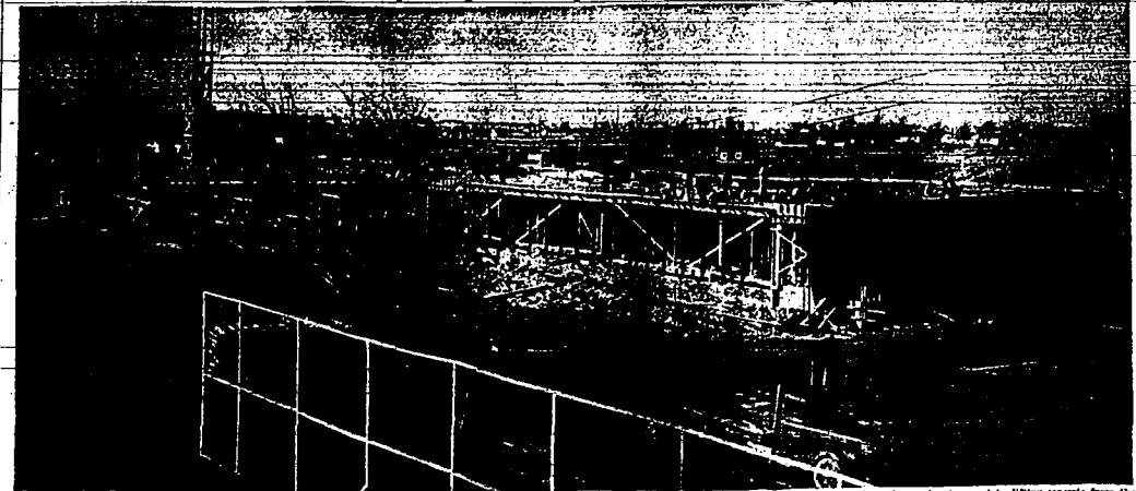
Photo above shows the new Twin Falls county hospital as it appeared Friday. Workers have just completed work on the "back structure" of the first floor for the five-floor building. Work was delayed earlier in the year when day excavations were found necessary for a solid foundation.
