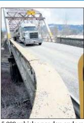
5,000 vehicles per day, and we don't envy the drivers. The bridge scored an outrageously low 'sufficiency rating' of 2 out of 100 in the National Bridge Inventory. Last year, a 30- by 30-inch piece of the deck was found hanging by its rebar."
