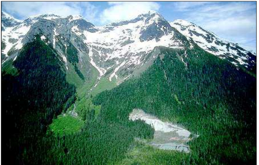
In this undated file photo by Coeur Alaska, the entrance tunnel and water treatment facility for the Kensington Gold Mine against Lion Head Mountain near Juneau, Alaska can be seen.
