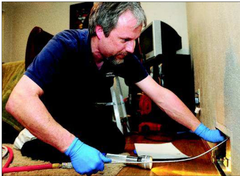
Gary Sipe, co-owner of Air Quality Services in Twin Falls, cleans out an air duct Thursday in Twin Falls.
