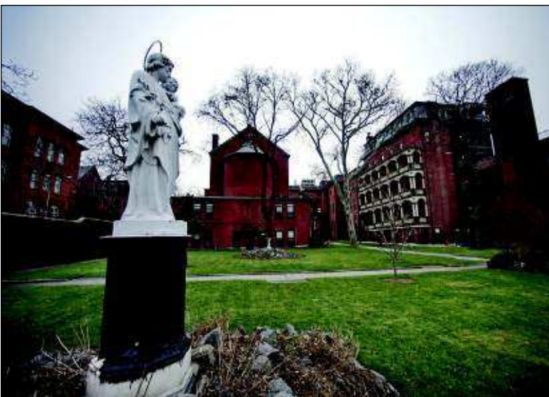
A preservationist group is seeking landmark status for the stately edifice of the Sisters of Mercy convent, designed by 19th century church architect Patrick C. Keely.
