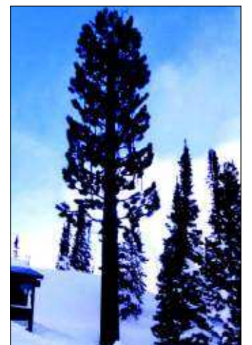
Photo courtesy Idaho Tower Co.
